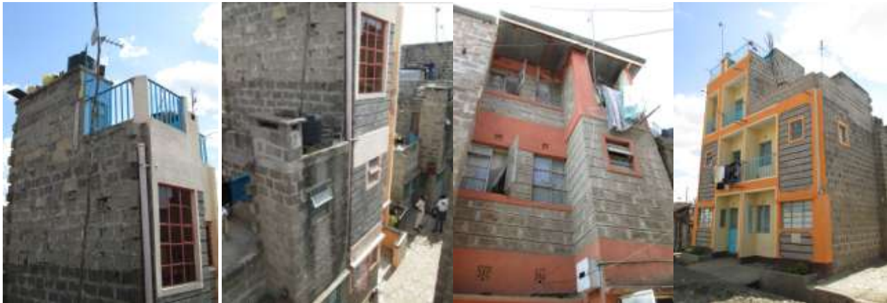
Fig. 7-8-9-10-11-12-13 Housing condition, internally and externally ( photo by Laura Burocco, September 2012 )
